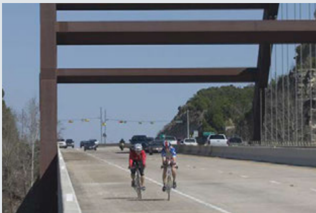
Pennybacker Bridge, Loop 360, Austin, TX
