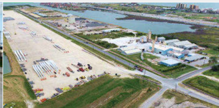
Port of Corpus Christi Rincon Road
