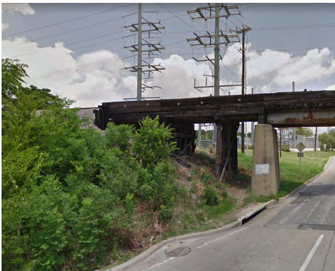
Figure 3-7: TRE Bridge over Inwood Road
