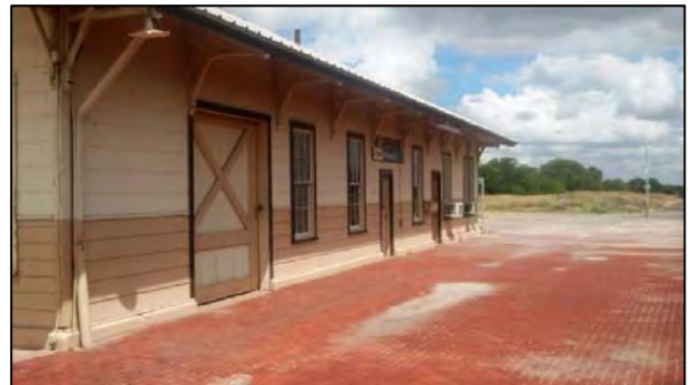
Figure 2-48: McGregor, Texas Station
