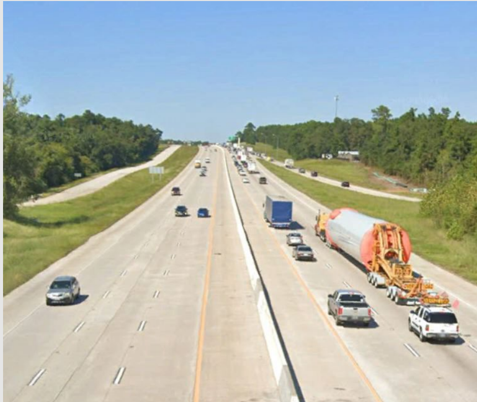
Example of Completed IH 45 Main Lanes
