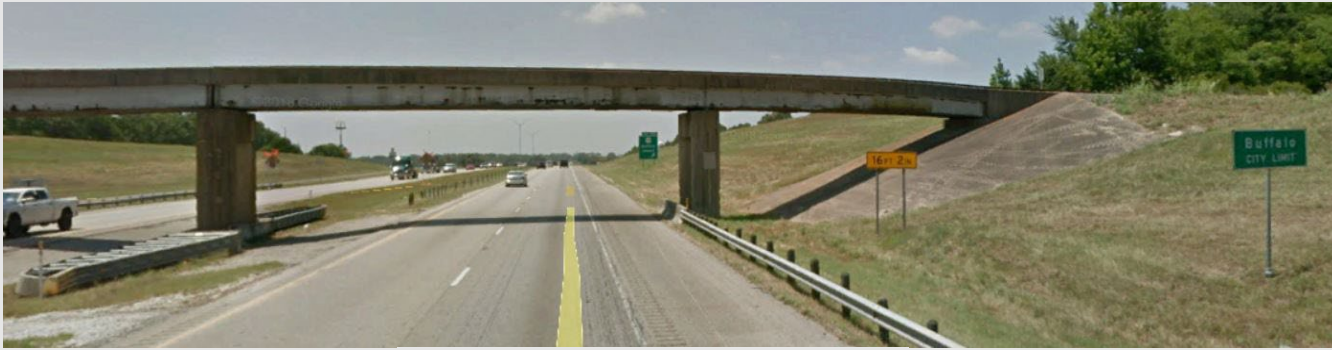
Example of low clearance/short span railroad structure
